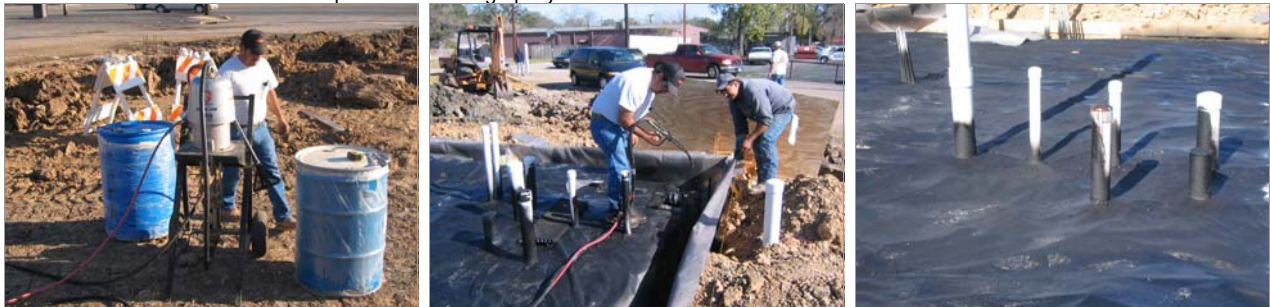
STEP 4: LIQUID BOOT® Gas Vapor Barrier being sprayed.
