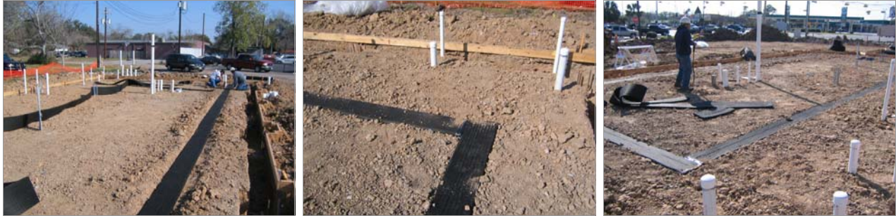
STEP 1: LIQUID BOOT® GeoVent being installed for the passive venting layer
