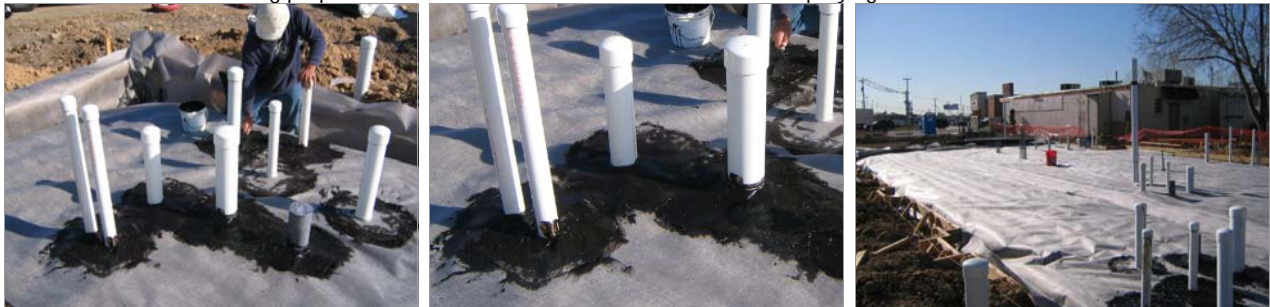
STEP 3: Penetrations being prepared with LIQUID BOOT® Trowel Grade before spraying.
